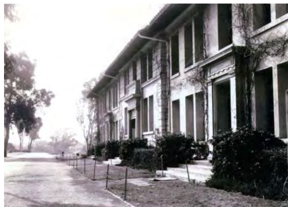
Main east façade with central and flanking entries.
