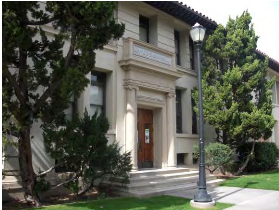
View of center entry on east elevation.
