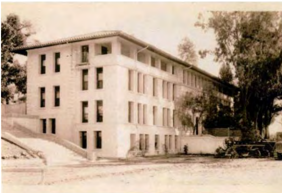
View from northwest showing stepped floors and sleeping porches
