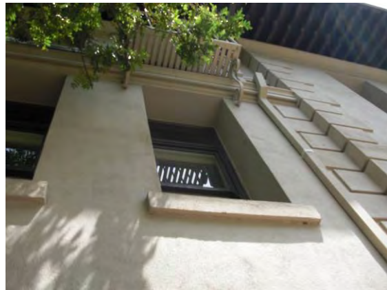
Original window sills, quoins and metal balconies
