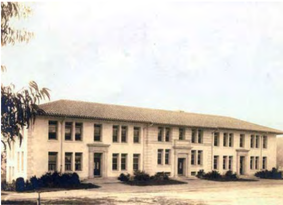
Early view of main east façade.
