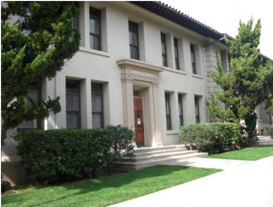
View of east elevation at southern entry.
