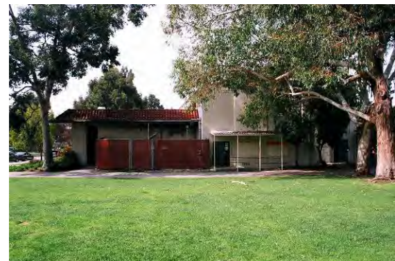
View looking west from Swan Hall at site for addition.
