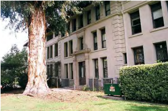
West façade with central entry portal.
