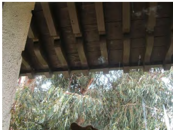
Roof eave detail with shaped rafters.
