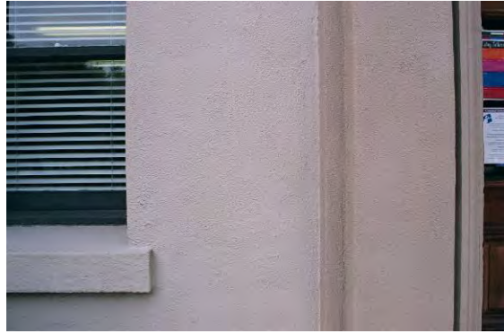
Exterior detail at window opening
