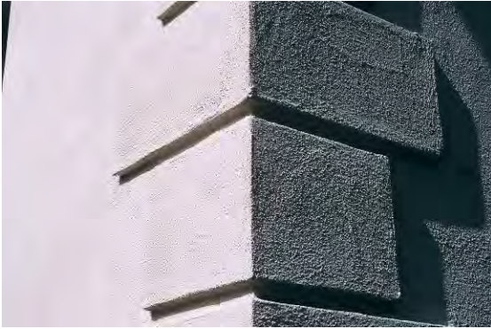
Exterior detail at corner plaster quoins
