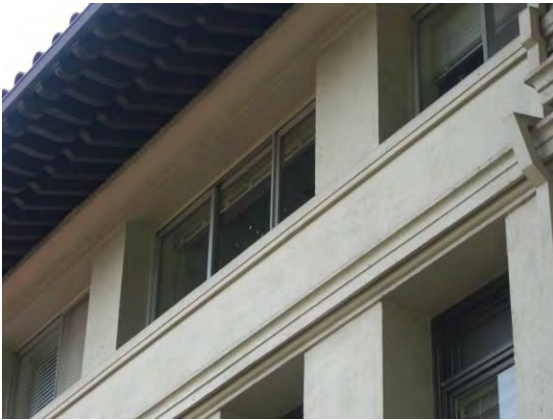
Windows at original sleeping porches
