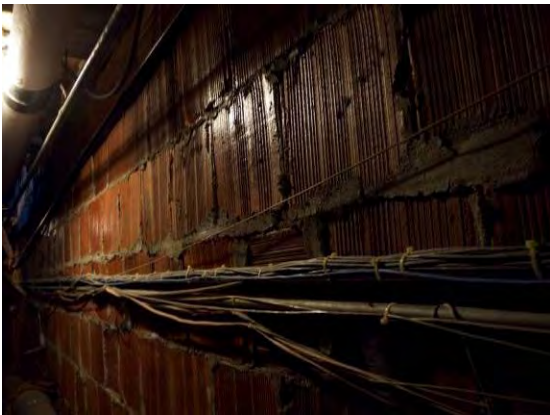
View inside HCT wall
