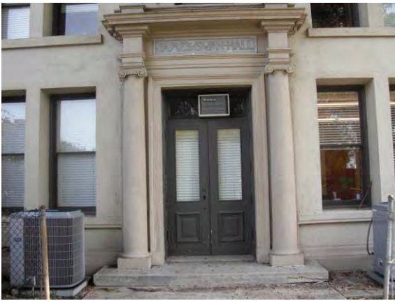
Entry on west with double doors and decorative surround.
