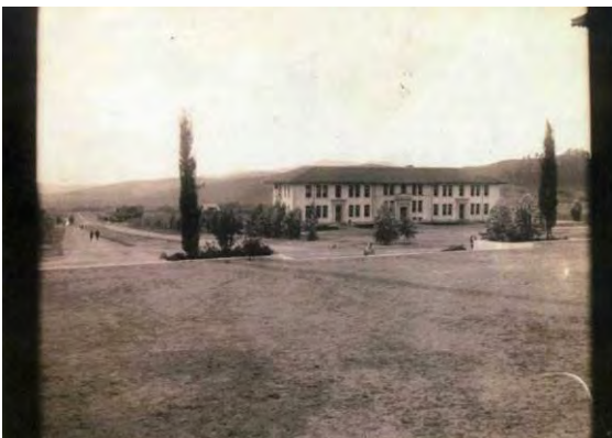
View of east elevation.
