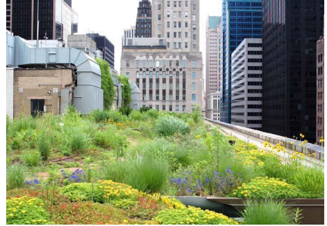
“Green roofs” use vegetation as a rooftop material to reduce heat gain and cool buildings. (Figure A.4.h)
