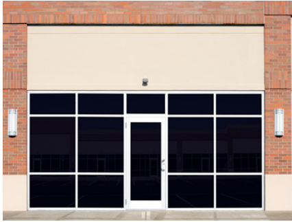
Dark and tinted windows along ground floor store fronts are uninviting and discouraged. (Figure A.3.vi)
