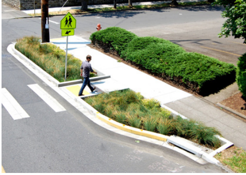
Curb extensions or bulbouts provide pedestrians both comfort and safety at pedestrian crosswalks. (Figure A.4.n)
