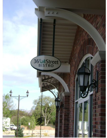
Signs should be deliberate and integrated as part of the building design. (Figure A.3.y)
