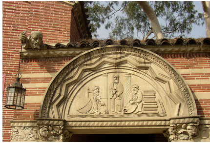
USC Mudd Hall Building (Figure A.2.p)
