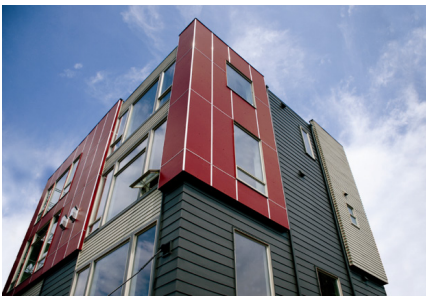
Use of Hardie Reveal Panels create a clean building façade. (Figure A.3.m)
