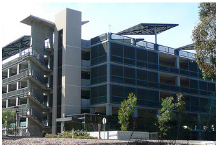
The tower of this parking structure highlights the entrance to both the stairway and elevator. There are also photovoltaic panels located on the top parking deck. (Figure A.3.e)
