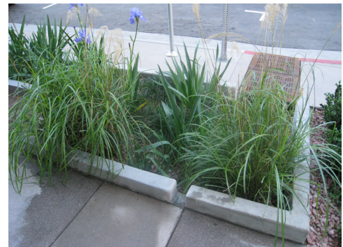
Details like the one pictured above, allows for the collection and cleansing of stormwater runoff. (Figure A.4.s)
