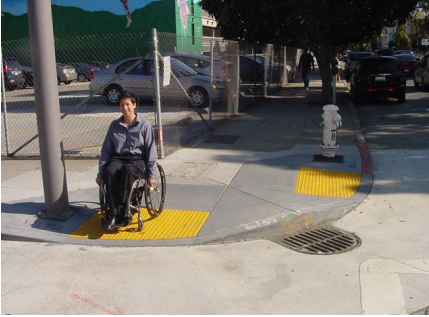
Dual sidewalk ramps that are directed to each crosswalk enhances accessibility for all users. (Figure A.4.p)
