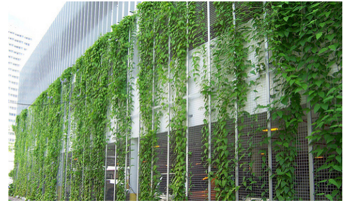
Landscaping features, such as the climbing vines shown above, are used to screen parking structures. (Figure A.4.r)
