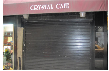
This roll down door is discouraged because it is not 75% transparent. (Figure A.3.r)
