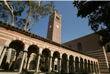
USC Mudd Hall Building (Figure A.2.g)
