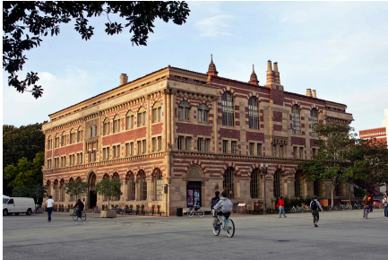
USC Student Union Building (Figure A.2.c)
