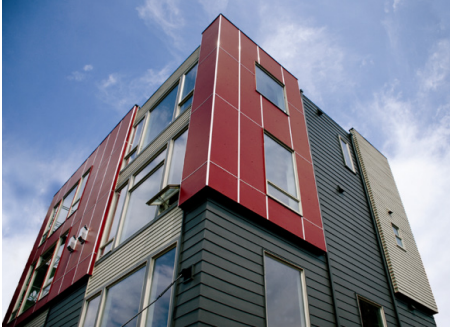
Hardie Reveal panels provide a finished architectural appearance and are encouraged. (Figure A.4.j)
