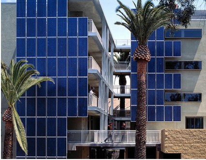
Integration of photovoltaic panels into this building's architecture contributes to a unique and sustainable design. (Figure A.3.l)
