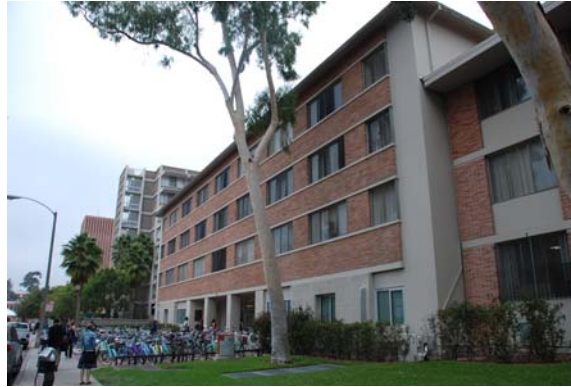
Von KleinSmid Memorial Residence Hall
