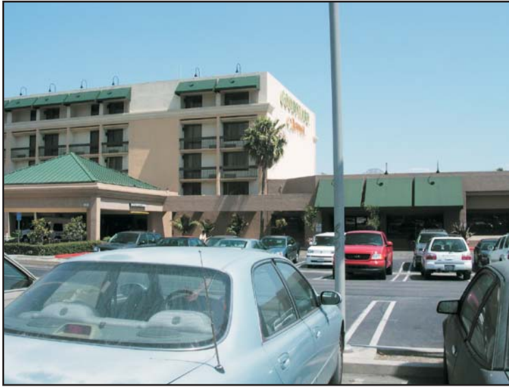
Photograph 5: View of the Marriott Courtyard Hotel and Cafe and Lounge building on the Add Area located south of the Mixed Use Project.
