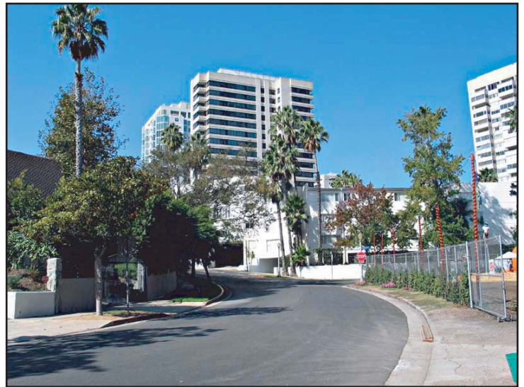
View 13: Looking west along Club View Drive towards the eastern side of the Beverly Hills Plaza Hotel. The project site is to the right, while single-family homes are to the left. Several high-rise condominium structures, including The Comstock, are visible in the background.
