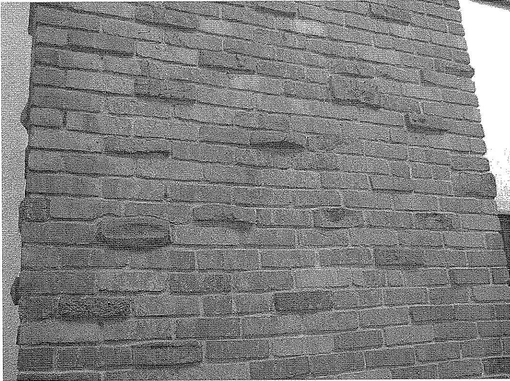
Oliver Flats, clinker bricks in chimney, 407-409 N. Orange Drive (Charles J. Fisher photo)
