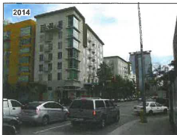
View 4: View from the intersection of the 9th Street and Flower Street looking northeast at the seven-story mixed-use development, 9th and Flower, constructed in 2007.
