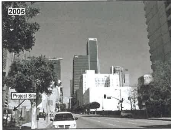
View 13: View from the west side of Flower Street looking north towards downtown Los Angeles.
