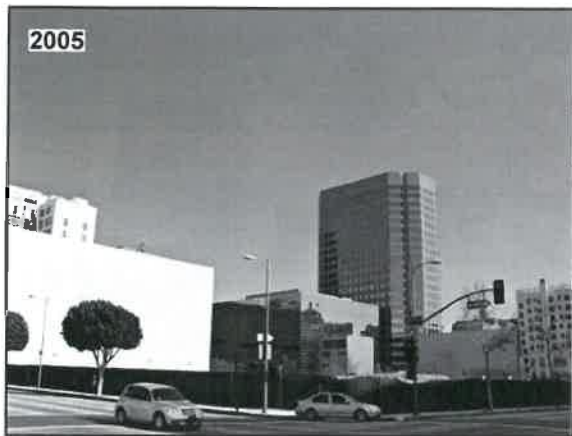
View 4: View from the Project Site looking northeast across the intersection of 9th Street and Flower Street towards a vacant lot under construction.
