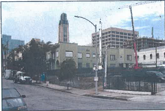
View 7: From the south side of Hoover Street looking west.
