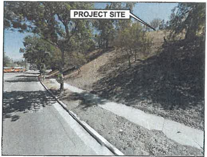
Photo B: View looking toward the northeast of the Project site.
