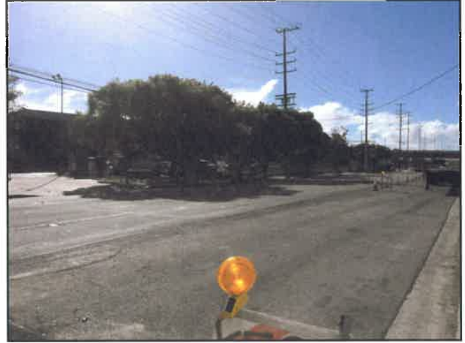
View 10: Looking south along Culver Boulevard.
