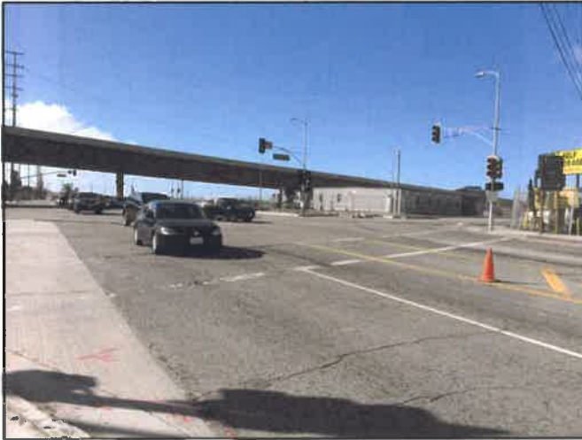
View 9: Looking south toward an elevated portion of the Marina Freeway.
